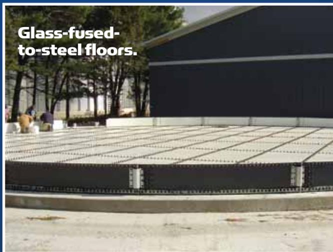
Nutristore features glass-fused-to-steel walls and floors. Floors are coated on both sides and will not corrode from the bottom.
